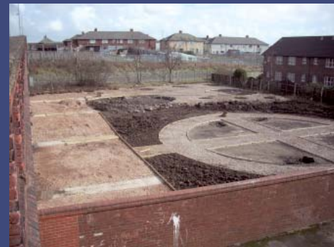
Construction progress April 2008
