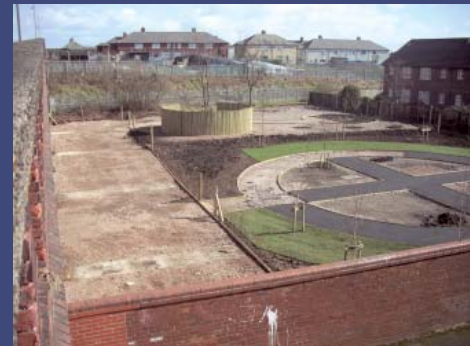
Construction progress June 2008
