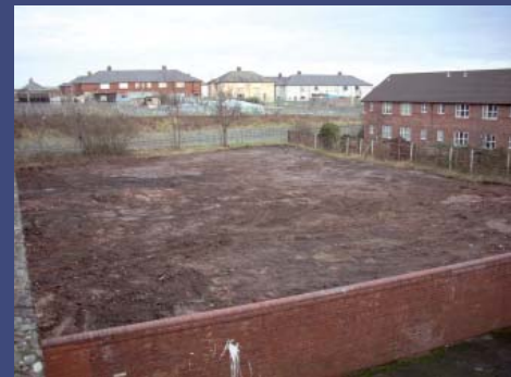
Construction progress February 2008
