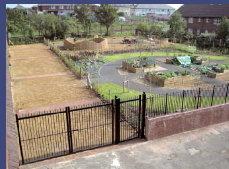
Nearing completion, including new fencing and gated entrance Sept 2008
